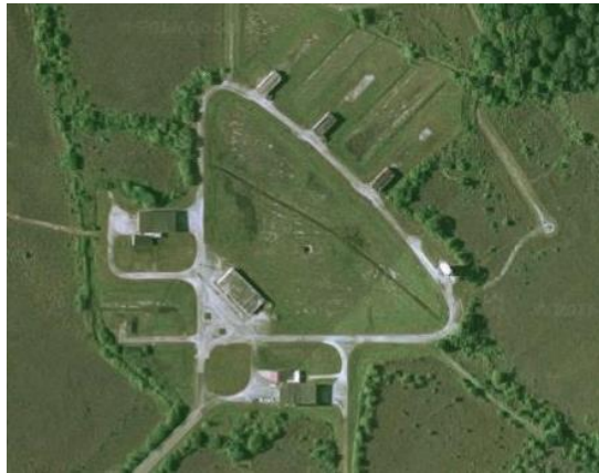
Figure 7: sounding rocket Site
