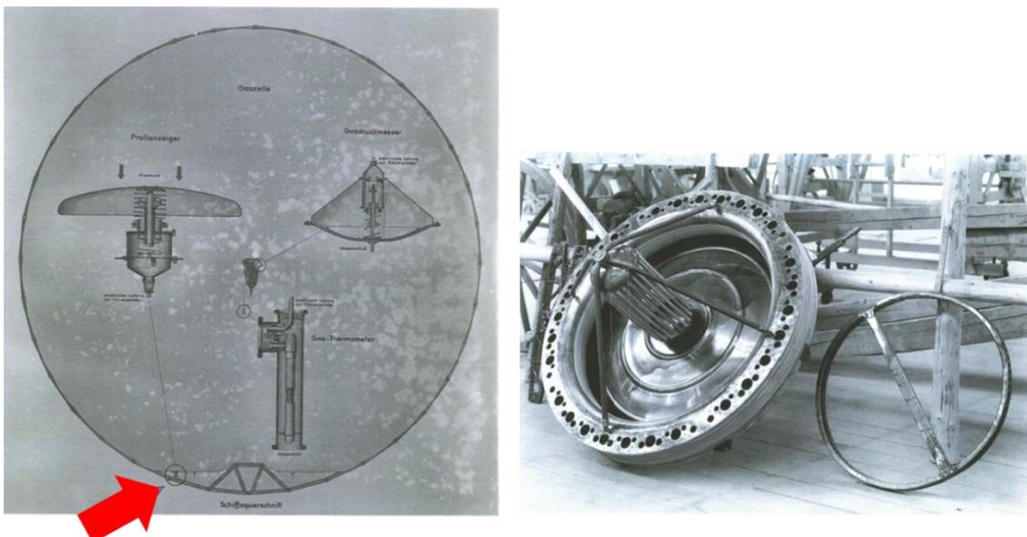
Figure 12: Zeppelin LZ-129 (Hindenburg). Overpressure sensor (left), Overpressure valve (right)
