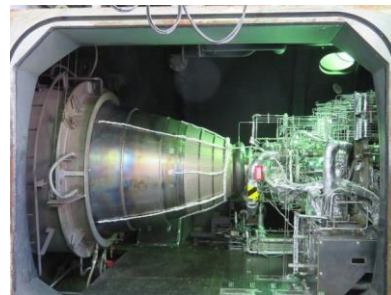
LE-5B-3 installed on HATS
