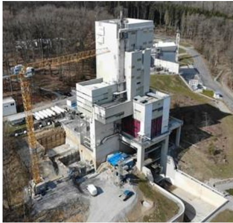
Fig. 4. aerial view of P5 during and after civil works (DLR Courtesy)
