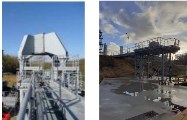
Fig. 7. Vernon PF20-B during building
