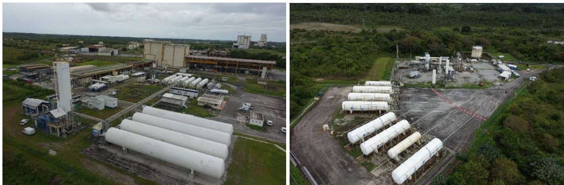
Figure 6: LOX and LH2 production plants at CSG
