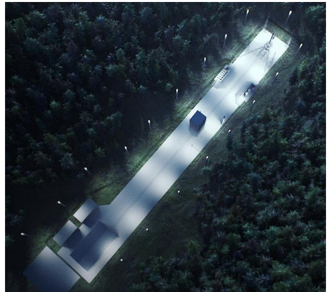
Figure 2 Launch Complex East; Reusability testing and Orbital launch
