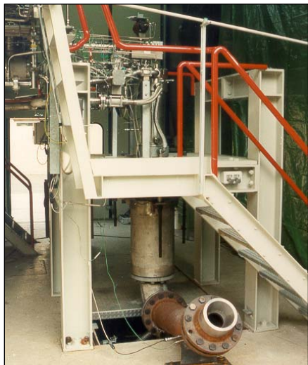
Fig. 2: Steam Generator Mode
