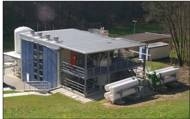
Fig. 5: P4 Steam Generator Building
