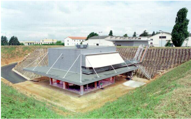
Figure 1: Martel Facility in CEAT
