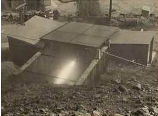
Fig. 4 Why it is called it a “Test Pit.” Firing 4.45-kN unit in Test Pit 3. (20 Feb 1942 JPL 383-236)
