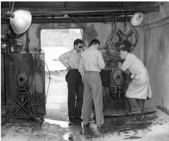
Fig. 6 Summerfield (r) with assistants Crofut and Powell in Liquid-Rocket Test Pit B testing the engines to be mounted in Douglas A-20A nacelles. (2 March 1942, six weeks before first flight on 15 April 1942) 27
